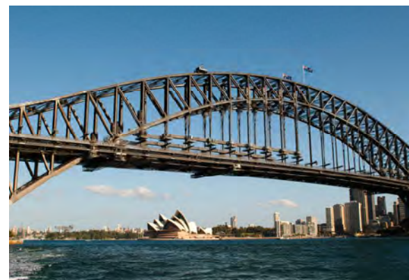
Figure 7.28 The Eiffel Tower in Paris and the Sydney Harbour Bridge were constructed using hot riveting.
